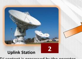
TV content is processed by the operator and then sent to the uplink station, where it is beamed up to the satellite.
