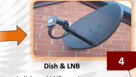
A dish and LNB receive signals from the satellite, which are then converted before being passed to the set top box.
